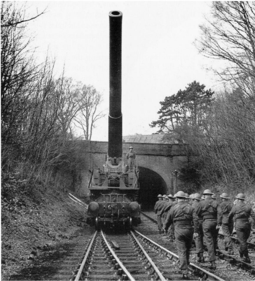
HMG Boche-Buster outside the south portal of Bourne Park Tunnel in 1941.
